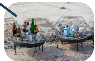
Bottle reefs on the beach prior to installation.
